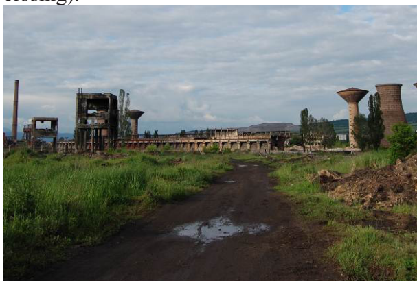
Fig. 8 Former coke-chemical plants area, contaminated soil before rehabilitation works
